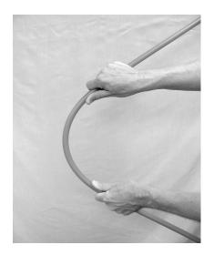
Measure and cut the pipe to length. Remember to allow extra length for expansion and contraction – PEX runs should never be stretched tight between fittings. A squeezetype PVC cutter will do a good job leaving a square and burr-free end. PEX can be bent into a fairly tight radius, but bend no tighter than a radius 6 times the outer diameter of the pipe.
